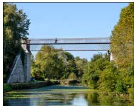
Footbridge in Arquennes - photo Greisch / JL-Deru
