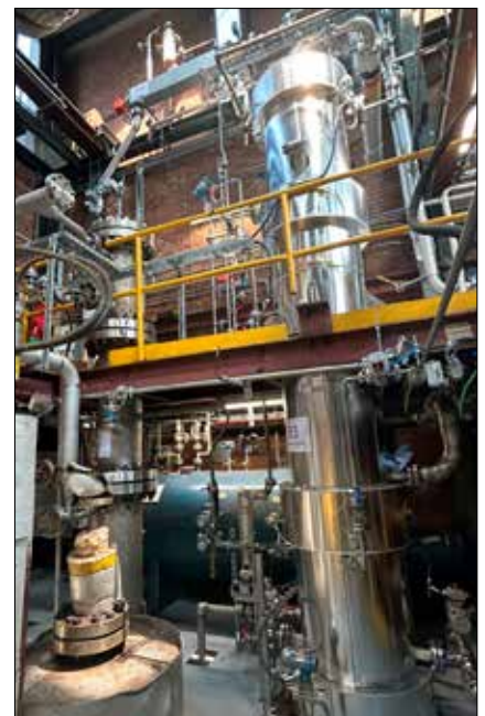
Fig. 5 - PiCaSSo pilot plant (1000 Nm 3 /h) for CO 2 capture by absorption
